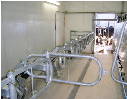
WALL CLADDING MILKING PARLOUR
